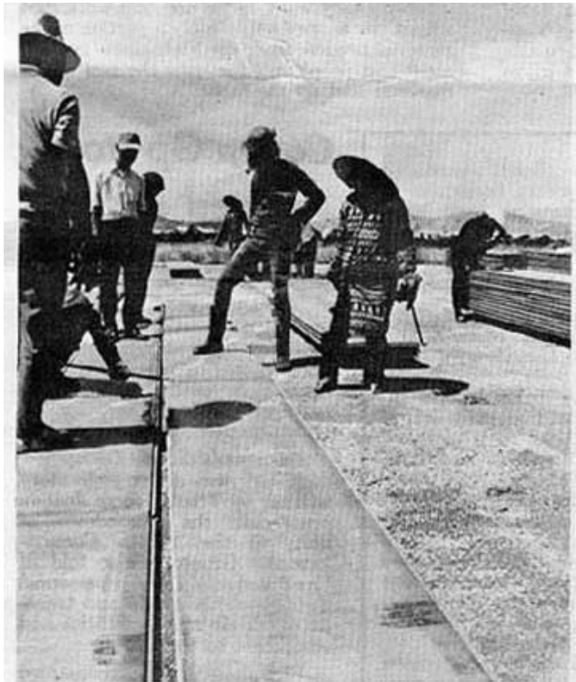
A 12-foot section of AM-2 aluminum matting is loosened by workers as Phan Rang's 10,000-foot long by 105-foot wide runway is dismantled for shipment to another base.
