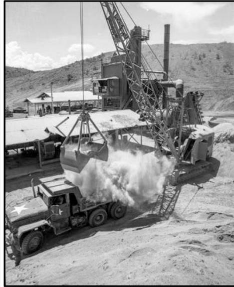
**Crane loading road base onto a dump truck.**
