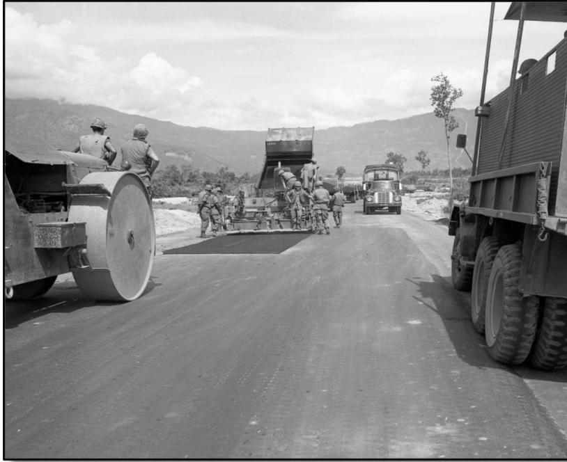
Army road crew laying down asphalt while the compactor waits.
