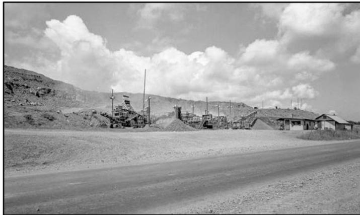
There was the crane operator who scooped up the crushed material and dumped it into the hopper to take it up to the top of the plant to a storage tank. Also the crane operator loaded road base into the dump trucks for deliver on site.
