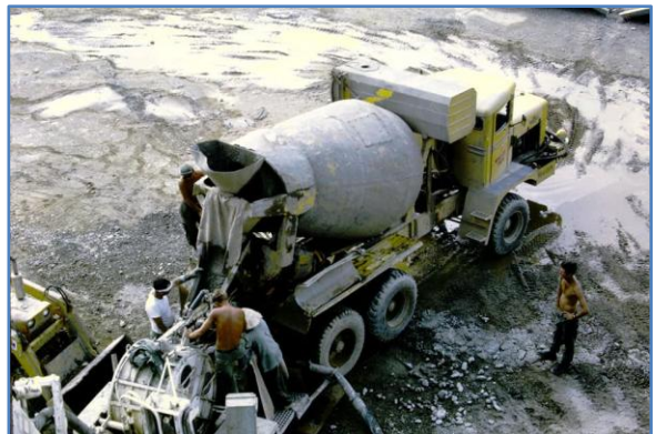
Concrete truck arrives at the construction site.
