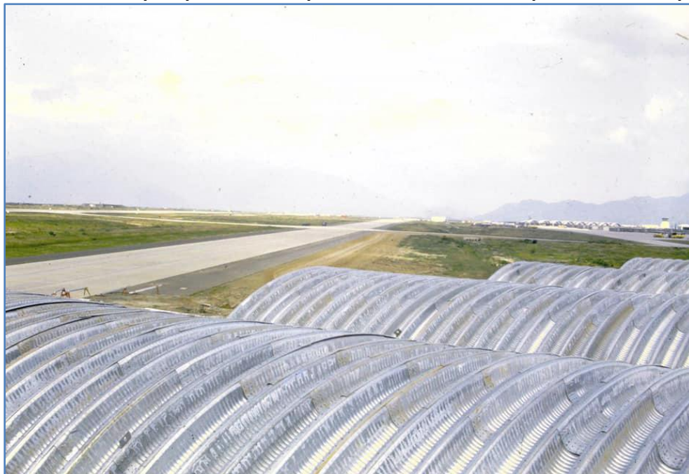
View from the top before concrete was poured.
