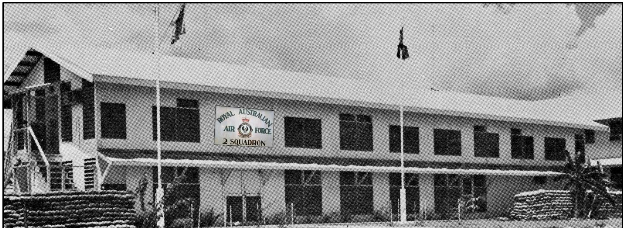
No. 2 Squadron Headquarters Building
